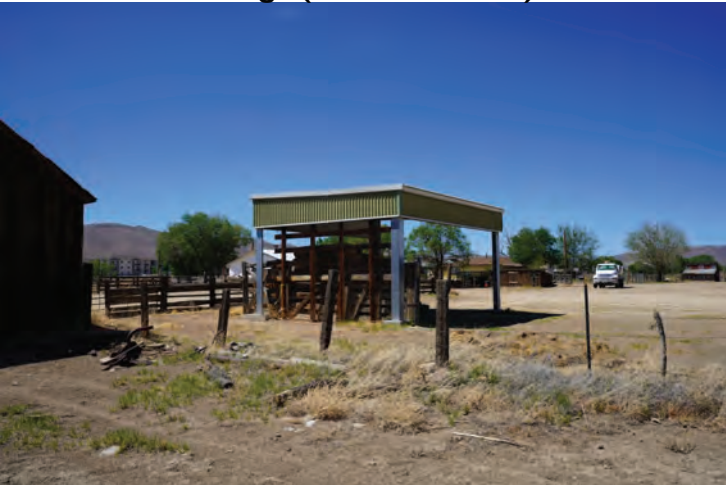
Hay storage structure
