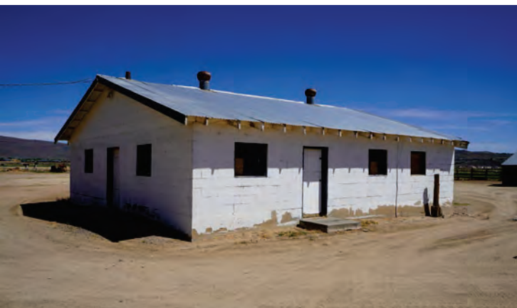
Old storage structure
