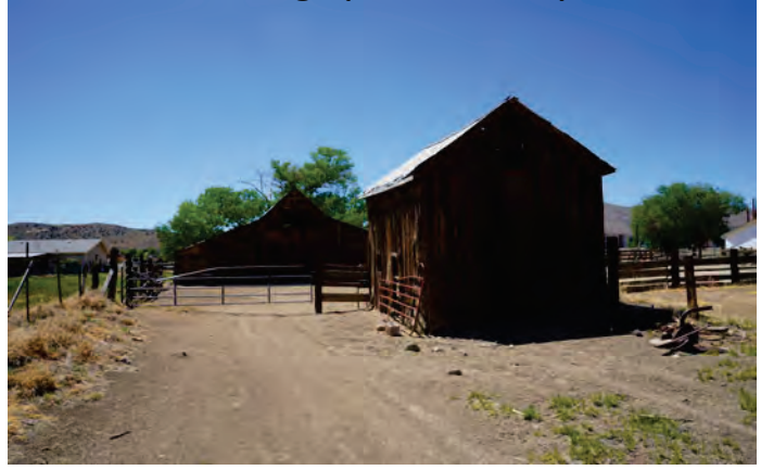
Old storage structure
