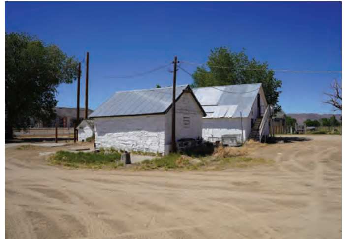
Old storage structure
