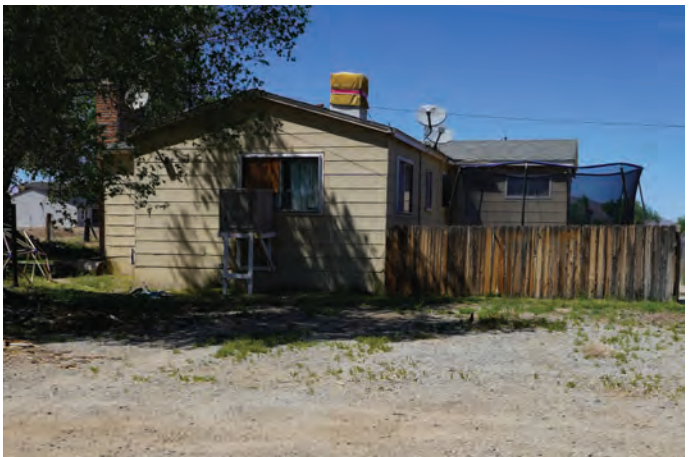
Private Residence II (south elevation)
