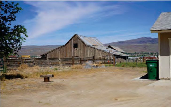
Old Barn for storage (west elevation)
